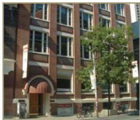
200 ADELAIDE ST. W. 4th Floor: 1,550 SF
